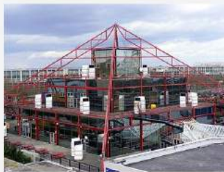
The Point multiplex cinema, Milton Keynes. Image source
