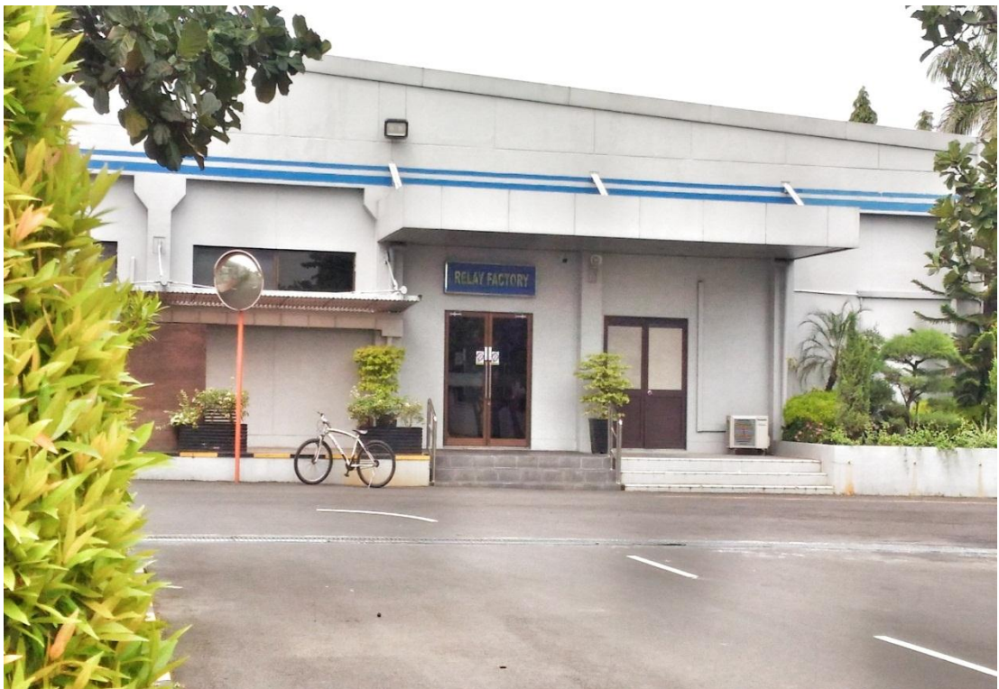
Figure 22 : Relay Department Building
