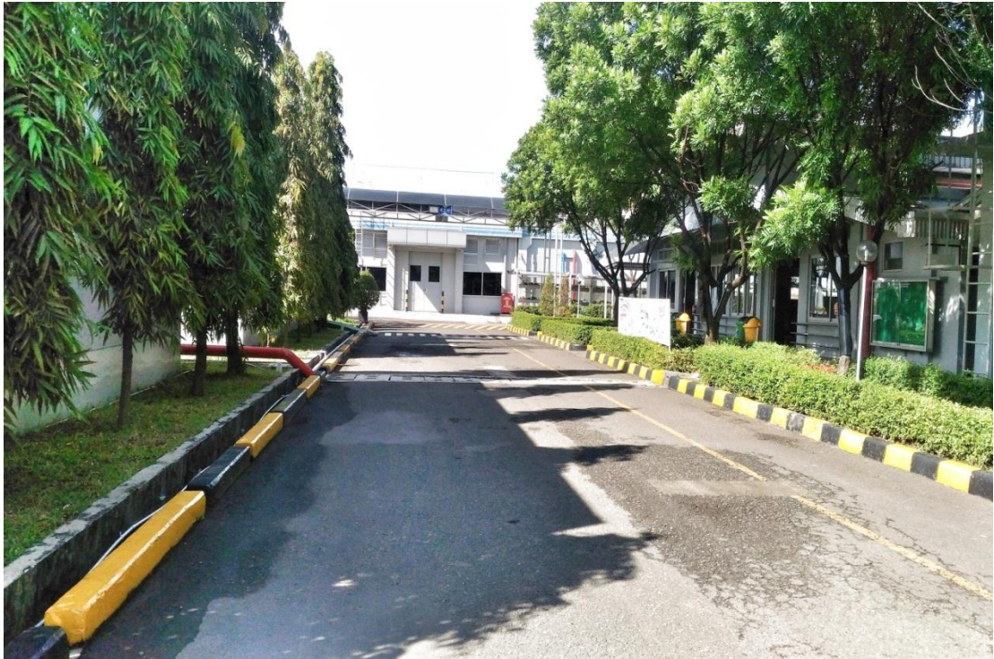
Figure 13 : Road Between Each Department Building
