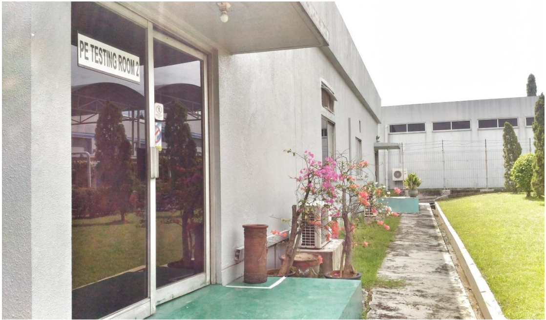
Figure 25 : PE Testing Room
