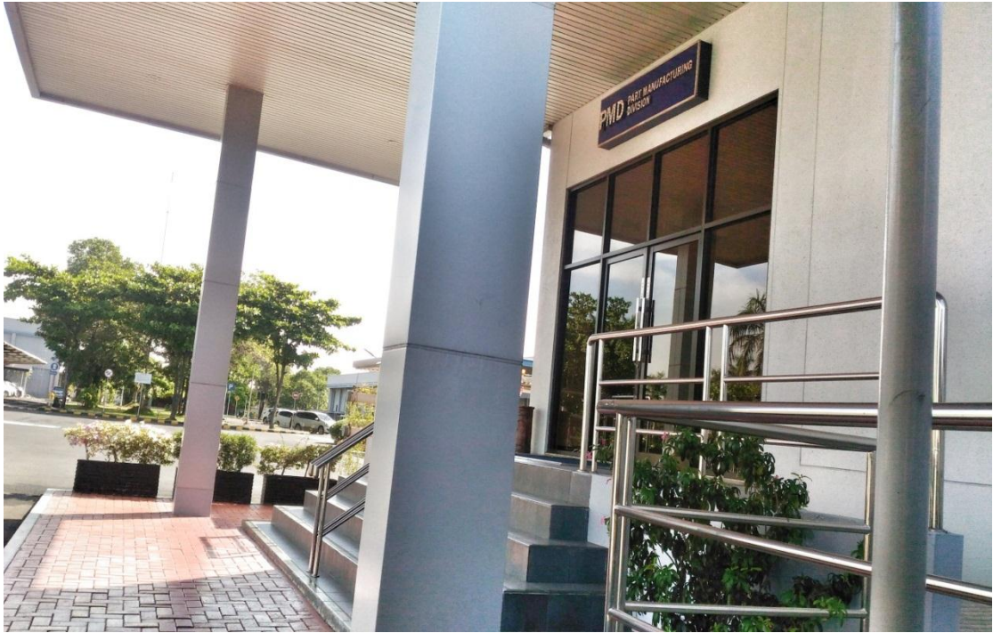
Figure 23 : PMD Department Building
